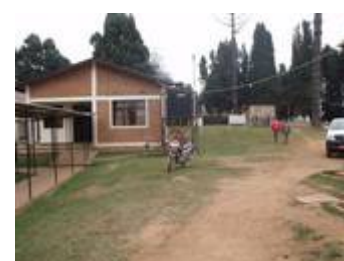
lack of security
